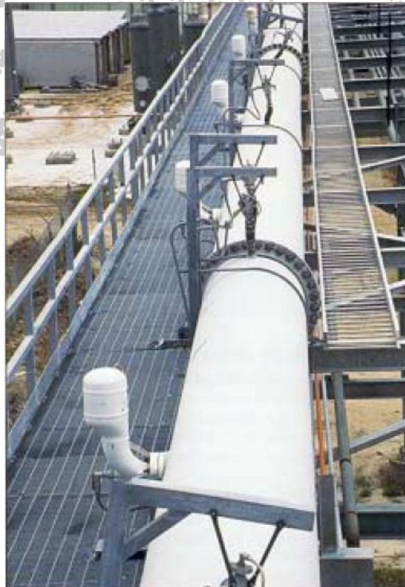
Explosion suppression system applied to pipeline
